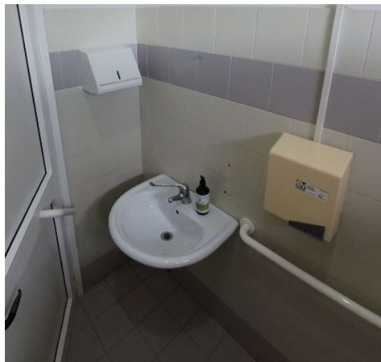
29. Accessible toilet interior
